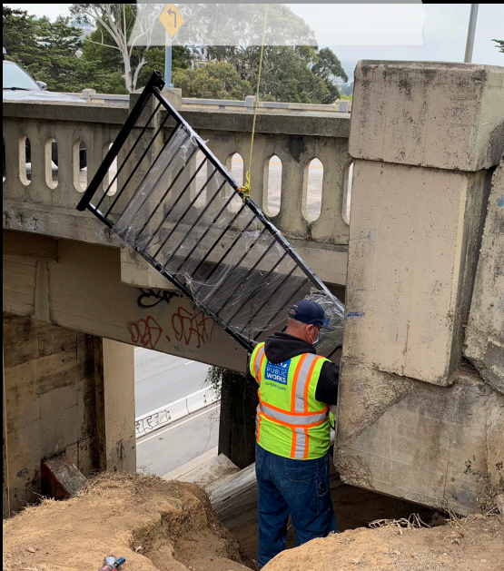
SHEET METAL CREWS INSTALL A BARRICADE ON THE RICHLAND BRIDGE.
