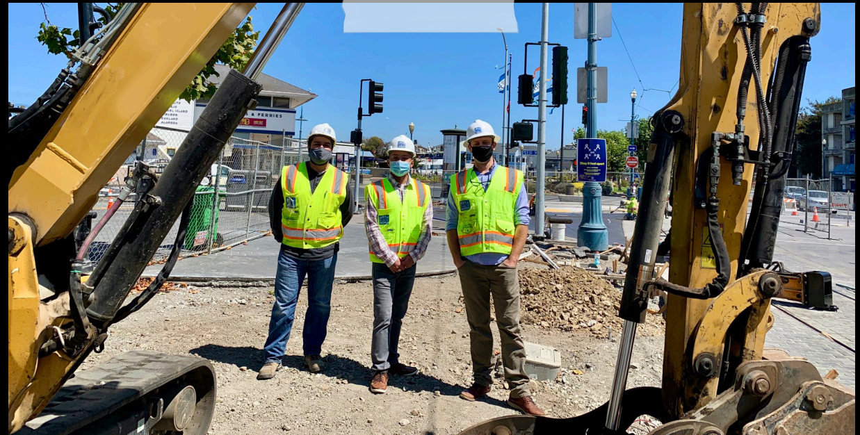
THE JEFFERSON STREETScape IMPROVEMENT PROJECT TEAM CHECKS ON CONSTRUCTION PROGRESS.
