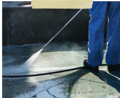
STEAM CLEANING: DEEP CLEANING & POWER WASHING GRIMY SIDEWALKS
