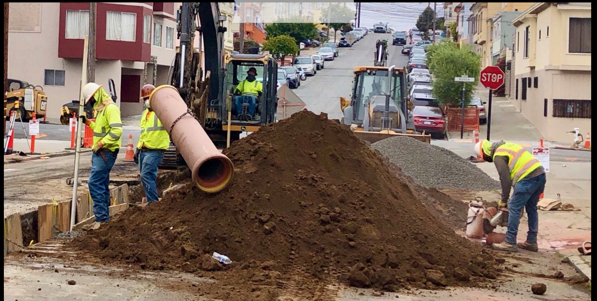
CONTRACTORS INSTALL A SEWER PIPE NEAR RUSSIA STREET.
