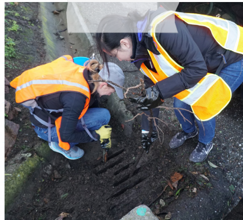
CLEARING LITTER AND LEAVES ATOP CATCH BASINS.
