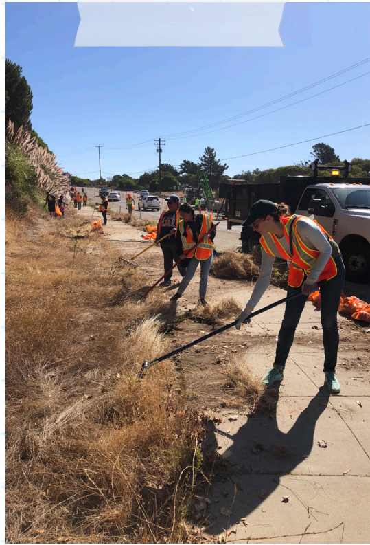
OVERGROWN WEEDS WERE REMOVED.
