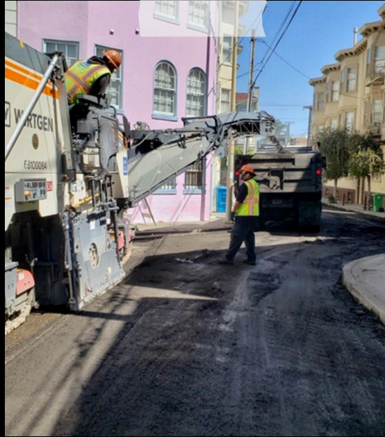
CREWS CONDUCT A ROADWAY GRINDING AND PAVING OPERATION.
