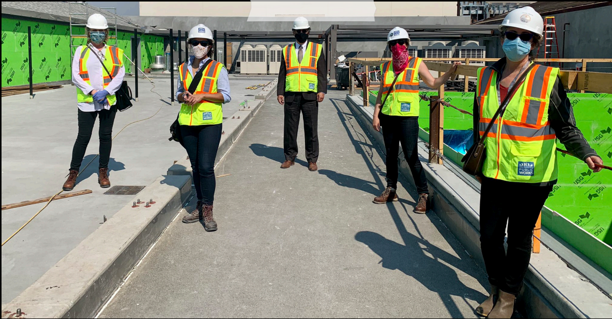
THE ANIMAL CARE AND CONTROL PROJECT TEAM STANDS ATOP THE CITY'S NEW ANIMAL SHELTER'S ROOFTOP TERRACE DURING CONSTRUCTION.
