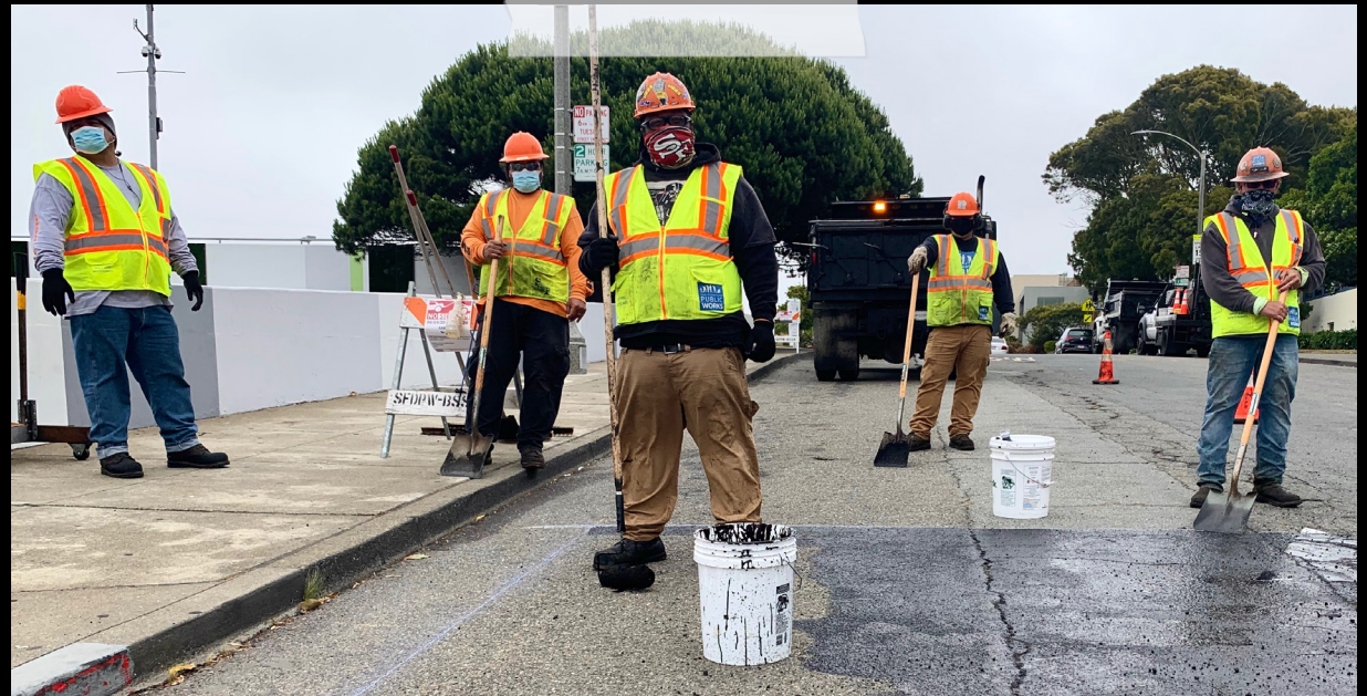
STREET REPAIR CREWS PROMOTE SAFE PRACTICES ON O'FARRELL STREET.
