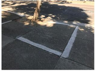
Sidewalk after being treated by concrete slicing.
