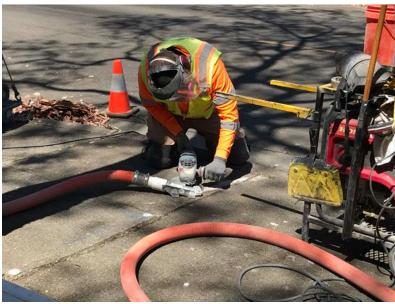
Concrete slicing is a fast, cost effective and environmentally friendly repair method that does not require removal and replacement of sidewalk squares.
